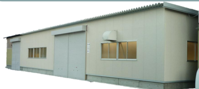
New building for transparent material development; September 2011
